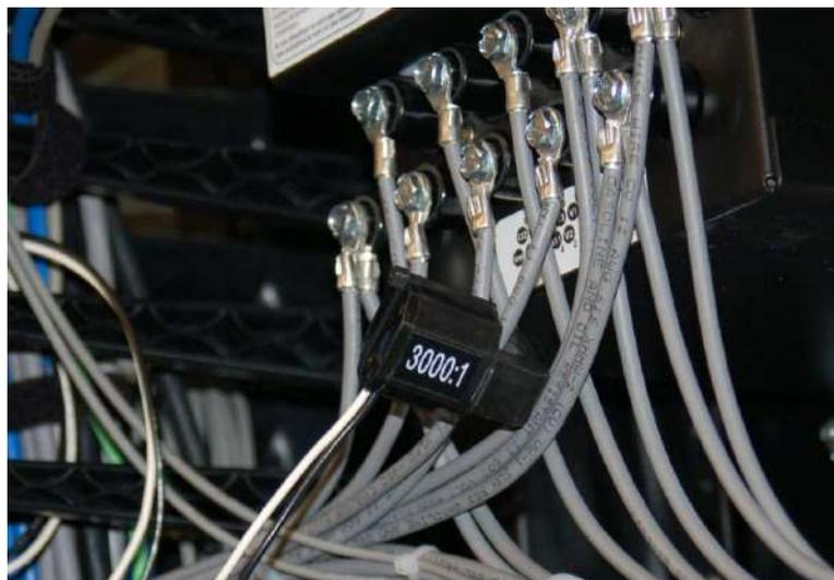
This CT's ratio of 3000:1 would step down a 5 amp AC signal to 1.667 milliamps AC.
