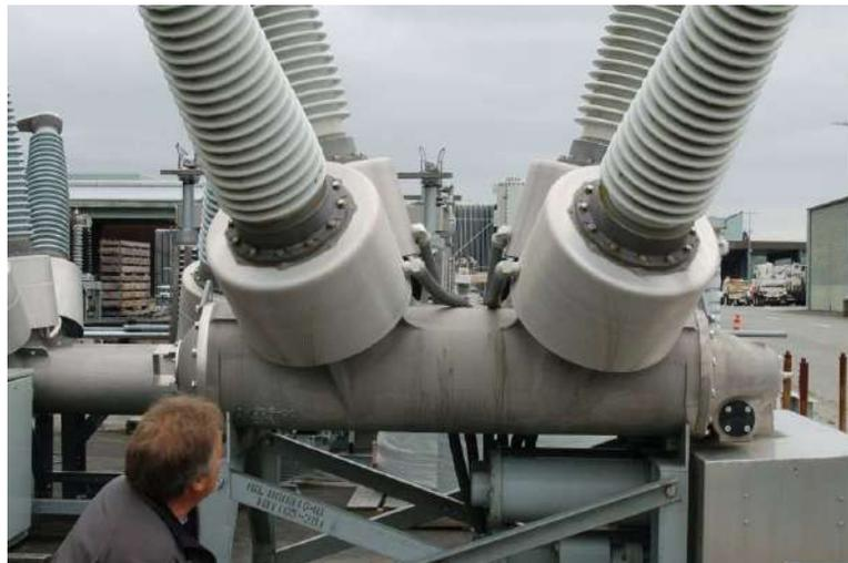
Signals from the bushing CTs on a circuit breaker may be connected to *protective relay* devices to trip the breaker in the event of any abnormal condition. If unused, a CT's secondary terminals are simply short-circuited at the panel.
