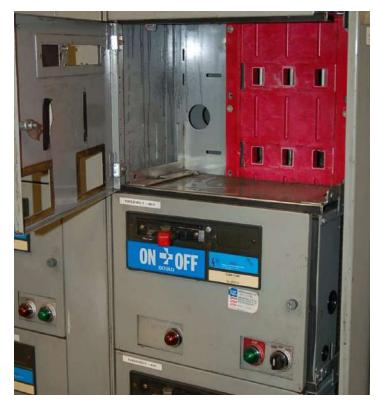
Industrial circuit breakers such as this are typically designed to be unplugged for ease of maintenance and replacement. If the "bucket" units are heavy, a lifting hoist is provided on the MCC to facilitate their removal and replacement.
