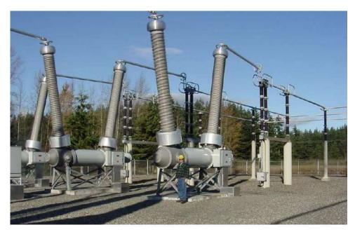
In this application, where three separate circuit breaker units independently interrupt current for the three-phase power lines, there is no mechanical link to synchronize the motion of the three contact sets. Instead, each single-phase circuit breaker actuates independently.
