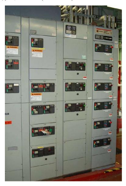
Note how each circuit breaker has its own on/off handle, for manual operation. These circuit breakers, like most low-voltage breakers, are capable of turning off ("tripping") on their own when
