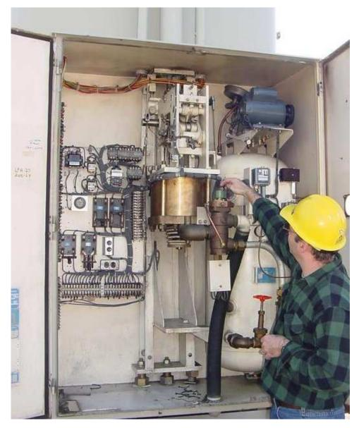
The man shown in this photograph is pointing to a solenoid valve designed to pass compressed air to and from the piston actuator. A large-diameter black hose runs from this solenoid through the bottom of the enclosure, allowing compressed air from the cylinder to vent to atmosphere.
