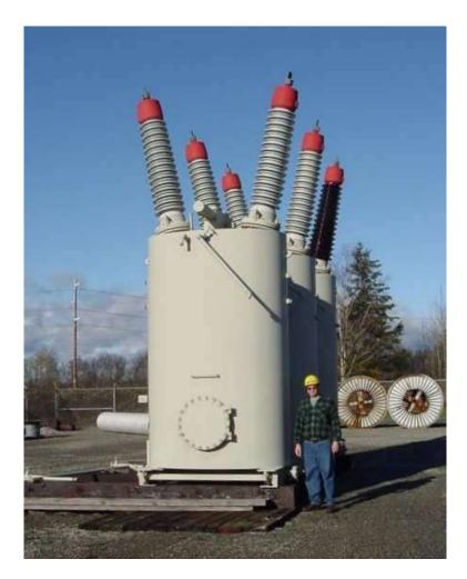
Each of the three circuit breakers (one for each line of the three-phase circuit) is mechanically linked by a common shaft at the top of the breaker tanks, so they all trip and close as one unit.
