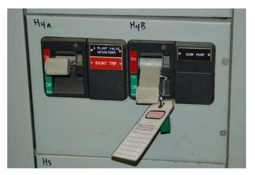
Note how the "Sump Pump" circuit breaker has been placed in the "off" position, its handle locked there by a padlock, a danger tag attached to notify any personnel of the reason for the breaker's lock-out.
