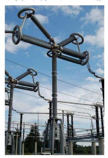
The actuating mechanism for this live-tank breaker is housed in the "can" assembly seen at the base, where the vertical insulator meets the steel supporting tower.
