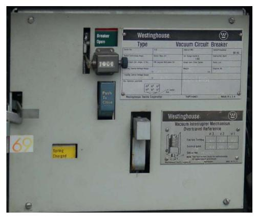
In this particular example, the actuating spring is charged, which means the breaker is in a state of readiness to switch from its present status (open, or tripped) to its opposite status (closed).
