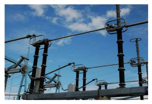
This particular high-voltage disconnect is motor-actuated, allowing all three disconnects to be operated in unison by remote control. When in the "open" state each metal arm points vertically toward the sky, clearly revealing its status to visual inspection. Lower-voltage disconnects are often built as manually-actuated devices, a crank handle or lever installed at ground level for a human lineman to actuate.
