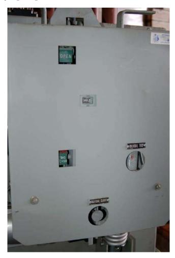
Green-colored flags seen on the front panel of this breaker show the contact status as "open" and the spring status as "discharged". This circuit breaker is incapable of any action until its spring is charged. Once the spring has been charged, pushing the button labeled "Manual trip" will cause the breaker contacts to open, and pushing the button labeled "Manual close" will cause the breaker contacts to close.
