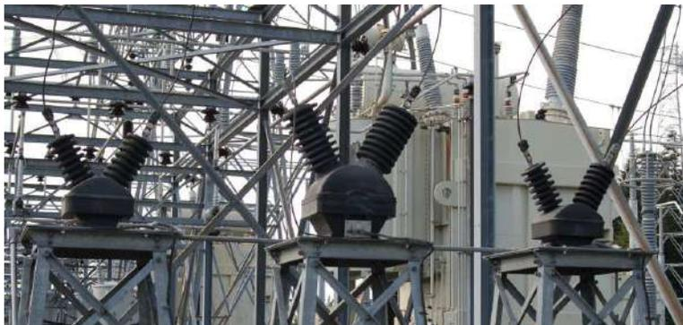
Another photograph of potential transformers appears here, showing three large PTs used to precisely step the phase-to-ground voltages for each phase of a 230 kV system (230 kV line voltage, 133 kV phase voltage) all the way down to 120 volts for the panel-mounted instruments to monitor:
